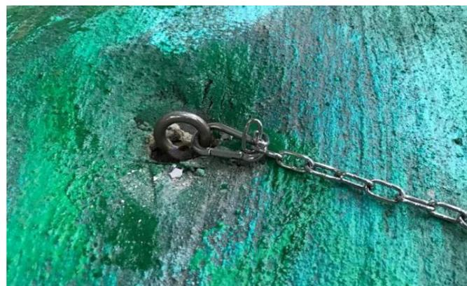
Figure 19. Anchorage point on the reef.
