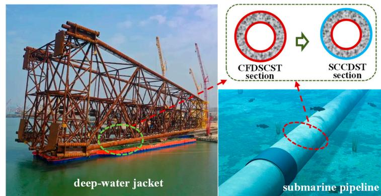
Figure 1. Potential engineering utilization of SCCDST members for avoiding corrosion.
