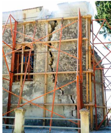
Figure 18. Damage at the N-W corner.
