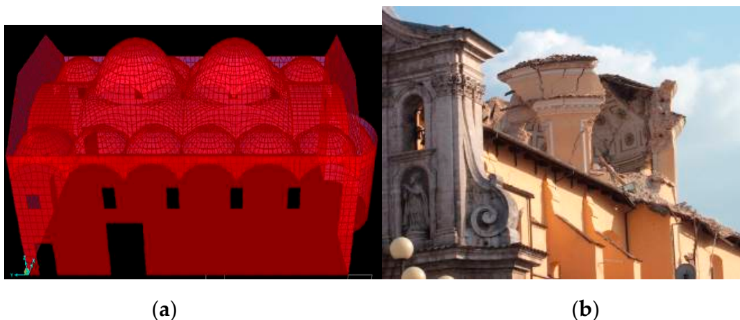
Figure 2. (a). Masonry vaulting; (b). Church of delle Anime Sante, L'Aquila earthquake 2009.
