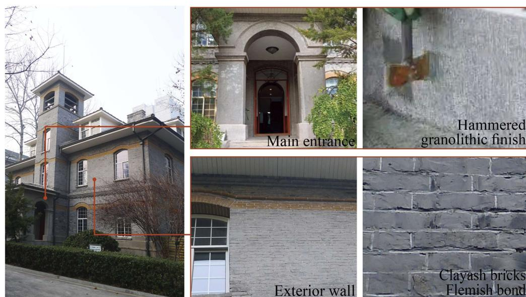
**Figure 12.** Materials and construction technology (source: author).
