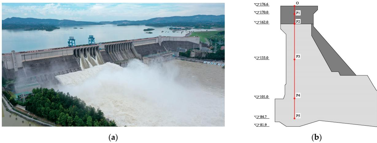
Figure 8. Overview of an actual project. (a) On-site graph; (b) plumb line layout of 13# dam section.
