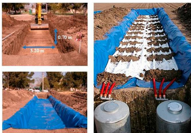
**Figure 1.** A lysimeter-like installation was set up allowing the recovery of the water drained from the 0.70 m soil profile and collected by draining perforated pipes placed along the bottom of each basin and connected to tanks located underground at the head of each field plot.
