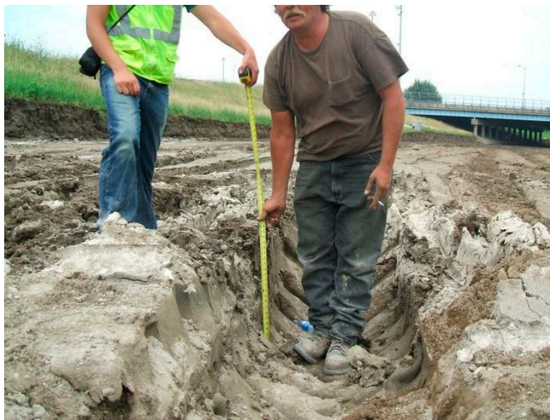
Figure 1. Failure of a weak soil subgrade due to construction traffic on I-75 Detroit, Michigan [2].
